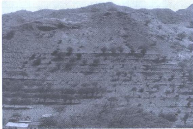
Figure 5. Slope treated with contour stone walls combined with agro-forest species— Achada Costa, Ribeira Seca.
