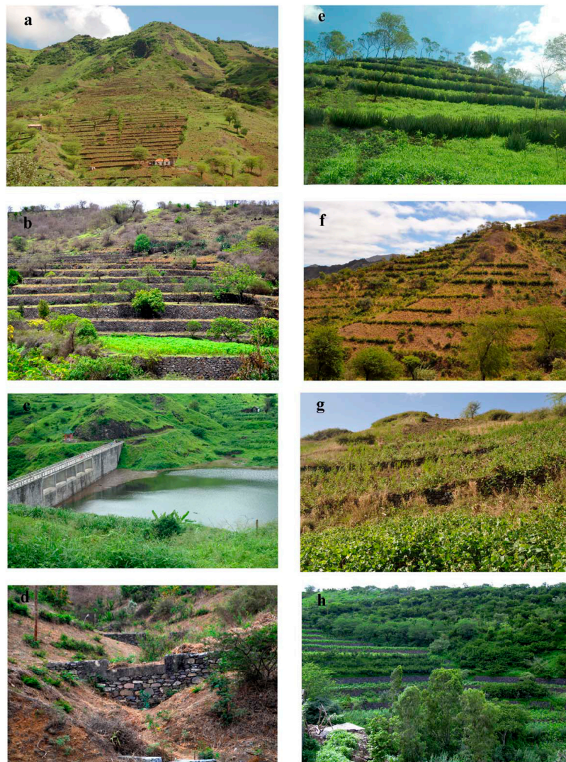
Figure 6. Vegetation and structural soil and water conservation measures in the Ribeira Seca Watershed: (a) contour rock walls; (b) terraces (São Jorge); (c) Water collecting dam (Poilão) during rainy season, d. check dams on water ways (Godim); (e) Aloe Vera barriers (São Jorge), (f) L. Leucocephala hedges (Godim); (g) Pigeon-pea on terraced fields; and (h) Afforestation with different species ( Longueira Baixo ).
